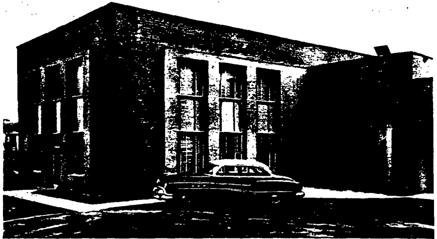
Offices, an auditorium, conference room and kitchen facilities are housed in the building. It is air-conditioned, of reinforced masonry with brick and concrete exterior, covers an area of 9,400 square feet. Offices are in the two-story wing at left, the auditorium is at the right.
